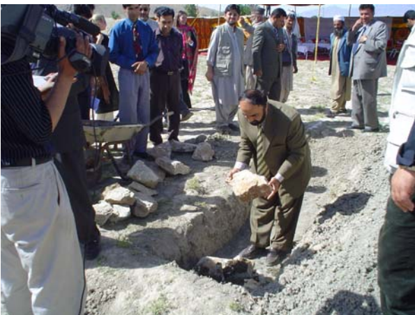
Dr. Karim Baz lays the ceremonial foundation stone for the BHF's generic medicines factory project during a Ground-breaking Ceremony in Kabul, June 2004.
